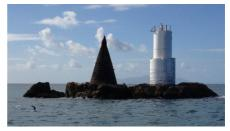
Maritime New Zealand's lighthouse expert says the white structure is the MNZ light, Admiralty number K3738 Flat Rock, originally built around 1918, and updated around 1950. The white tower is fibreglass, mounted on a round concrete pier. Its signal is a <u>white flash</u> <u>every seven seconds</u>. The dark stone spike is or was the original mark on the rock, probably pre-1900.
